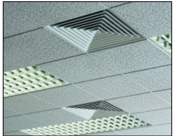
Louvre face diffusers in a typical installation
