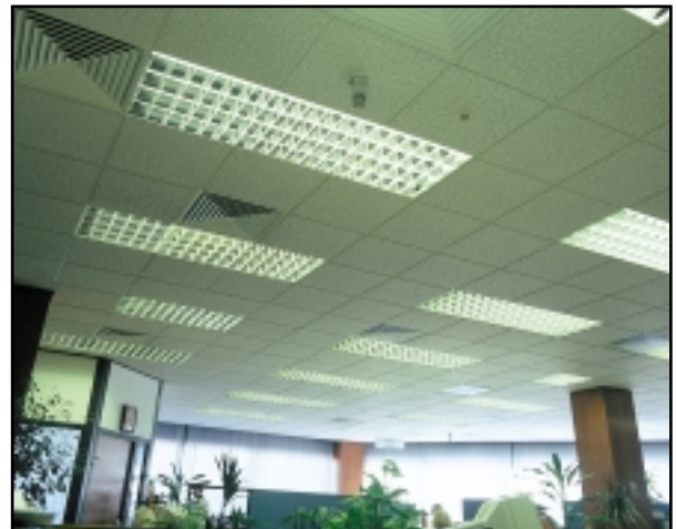
Louvre face diffusers in a typical installation
